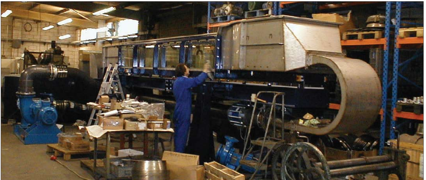
Loughborough University flume during construction.
